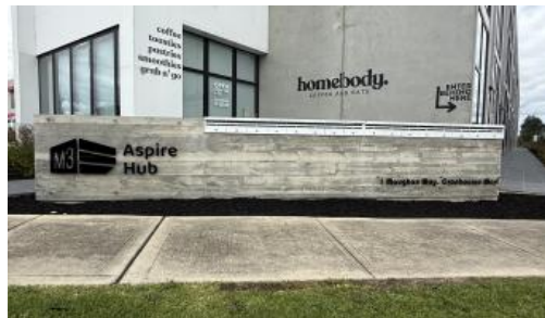
19 Maughan Way, Cranbourne West
